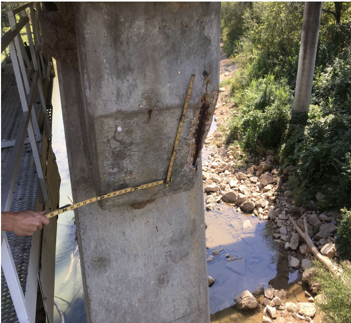
PHOTO 1 Description Spall with exposed rebar at the right cap haunch of pier #3.
