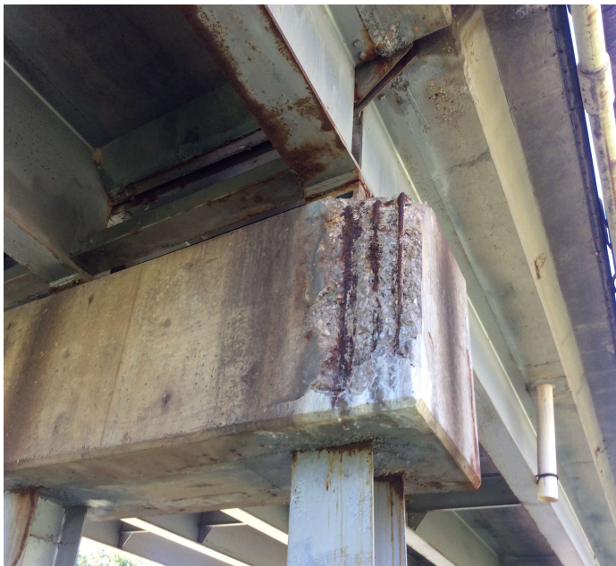
PHOTO 1 Description Spall with rebar exposed at left cap end of bent #3
